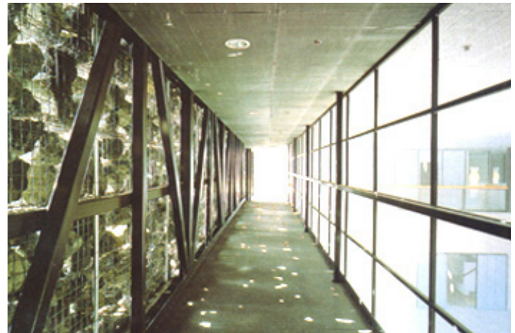
fig. 4 - Upper level walkway between the offices and tank room.
