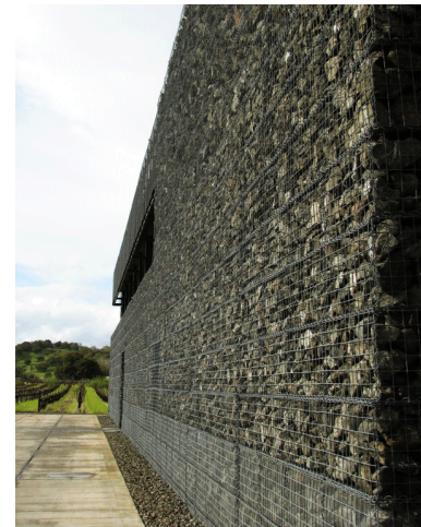
fig. 4 - Close up view of the gabion system.
