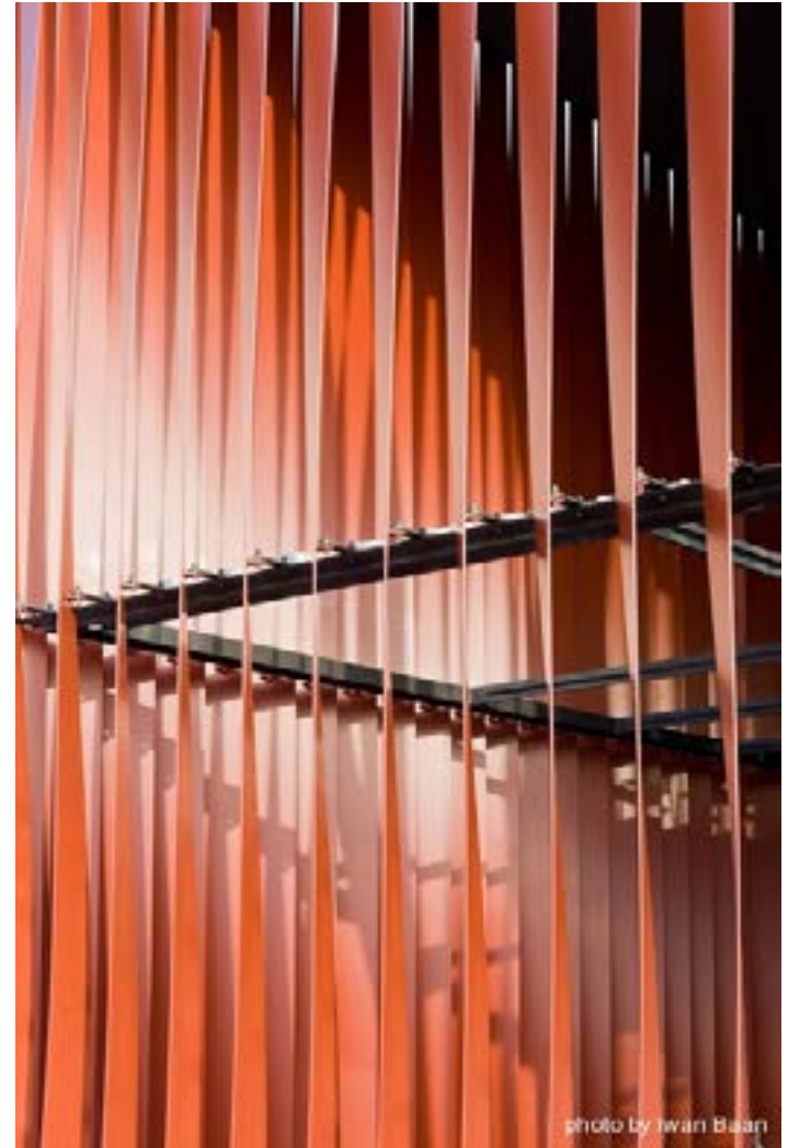
fig. 3 - Steel Ribbons Detail
